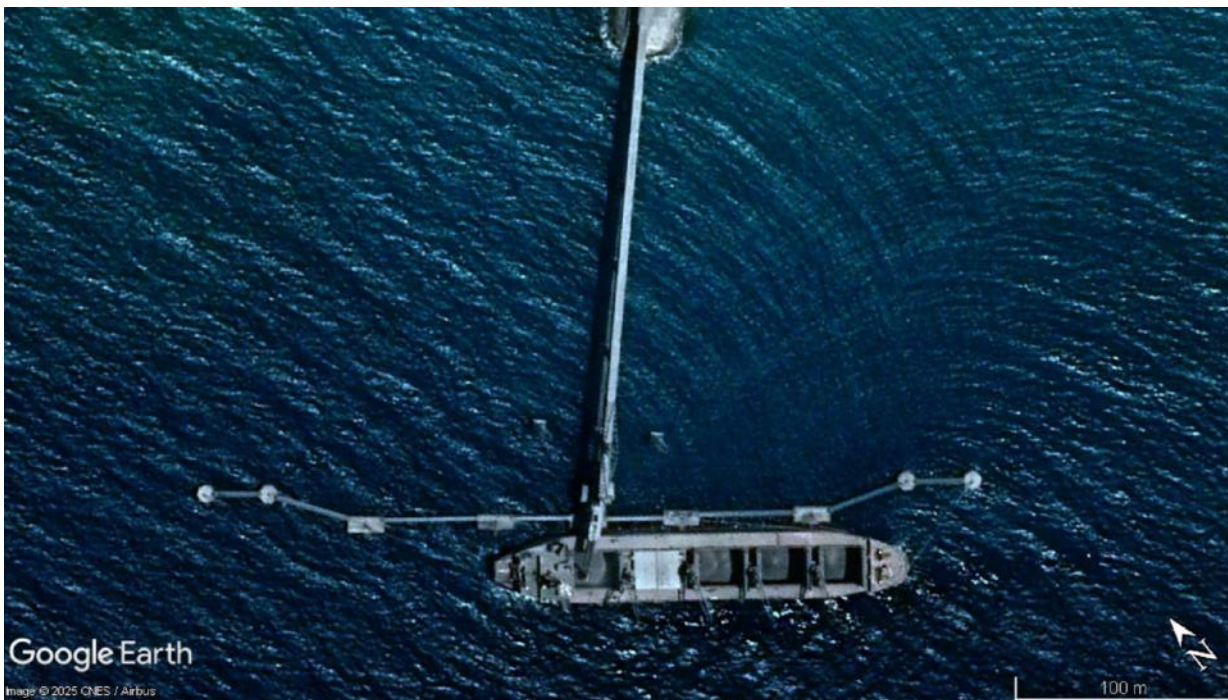
GOOGLE EARTH IMAGES OF JETTY
